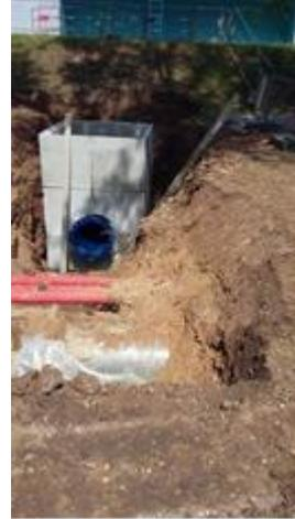
Raccordement hydraulique DN900 /regard
